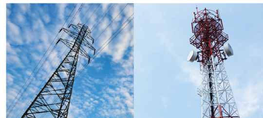
Radio & Electrical Towers
